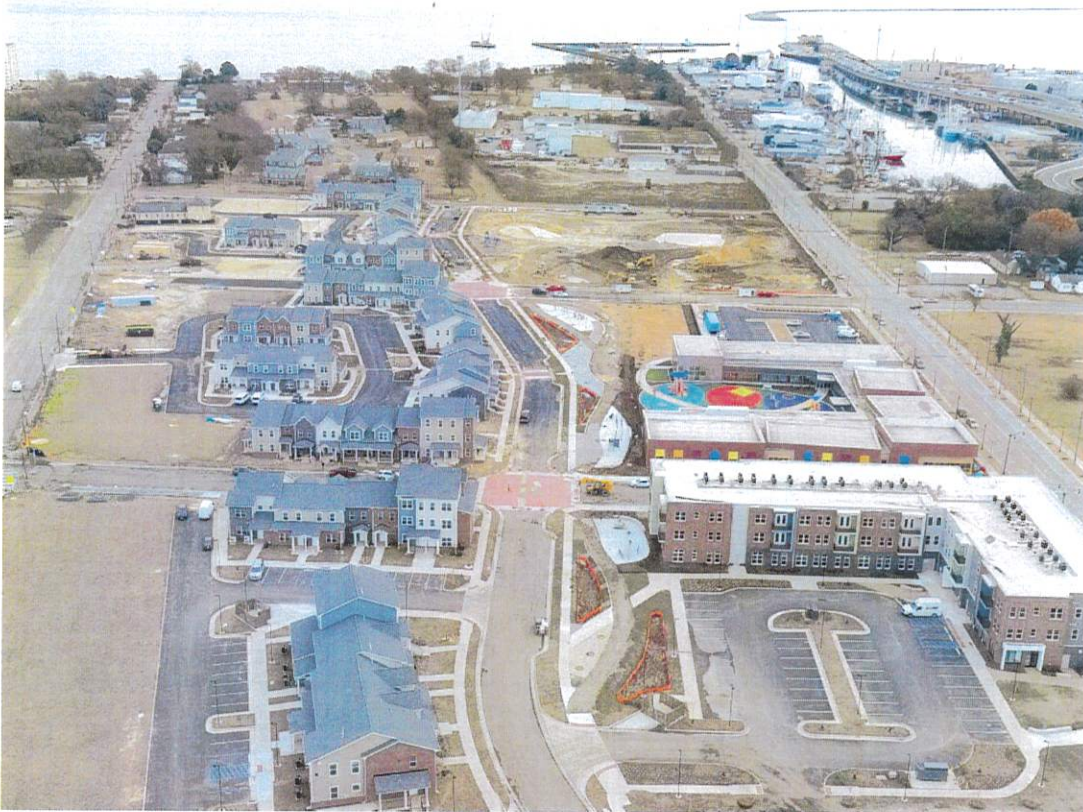
Construction at the former Ridley Place site – Legacy Landing
